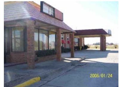
Building is Adjacent to 48 room Motel
