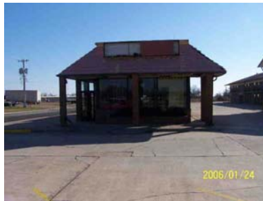
Front of Building
